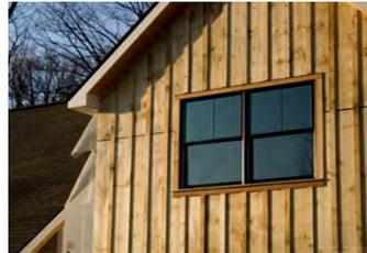
F14. As a major contributor to the feel and character of the street, wood – particularly Red Cedar, is the preferred material for exterior cladding. The use of cedar shake or shingle applications is especially favoured. Cedar lap siding and vertical board-and-batten are also preferred.
